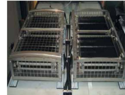
Stainless steel is also used for bolts, nuts and washers. The resistors are designed to avoid disturbing noises caused by pulsating current.
