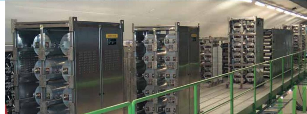
Braking Resistors for large motors are customised to best comply with any requirement: we have developed special Braking Resistors for important research institutes (among them Max Planck Institute) and for energies in excess of 3400MJ.
