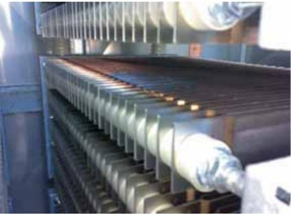
Starting and Braking Resistors are widely employed for controlling motors during start and/or stop.
