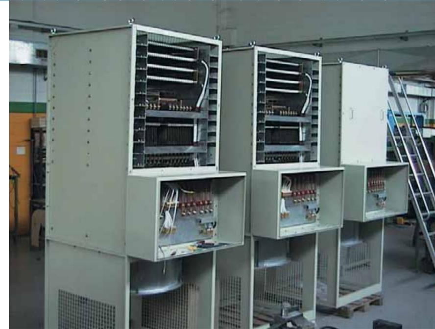
Microelettrica Load Banks can be controlled either locally or remotely (on request), through switches and contactors (also produced by Microelettrica).
